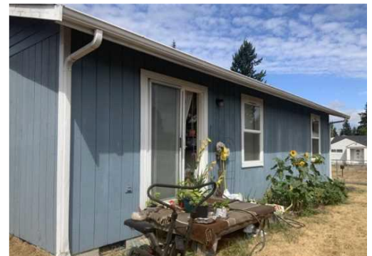
1 - LIPH #109 in 2021, located just south of the old PCHA Main Campus in Parkland.
